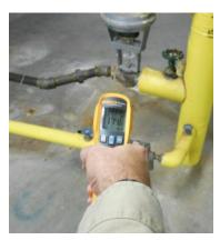
Viewing the temperature of the condensate line from a steam trap, to make sure it is functioning properly.
