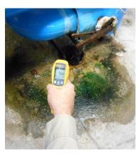
Taking the temperature of condensate as it goes into the drain
