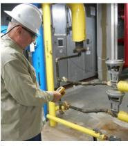
Testing the steam trap to see whether the trap has failed open and is wasting steam.
